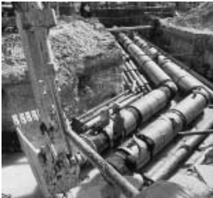
FOAMGLAS® insulation's excellent compressive strength permits direct underground burial.
