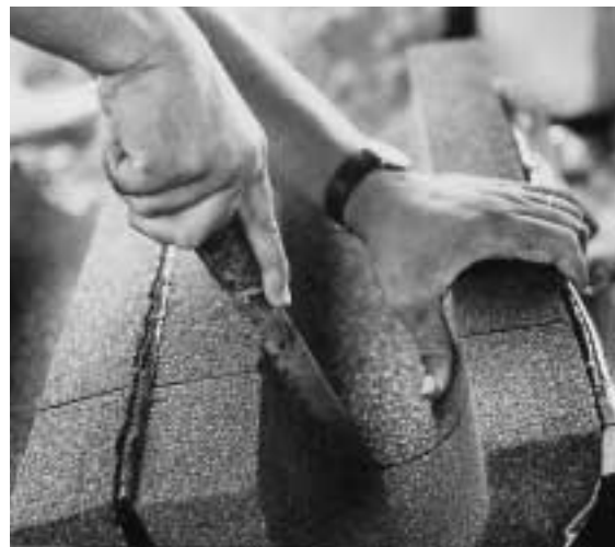
FOAMGLAS® insulation is easy to cut and shape with normal hand tools.
